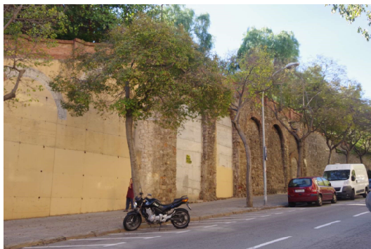
Vista general murs i obertures
