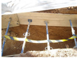
Rasa 1 Tram final entibat 2
