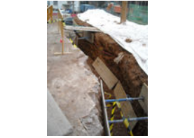
Rasa 1 Tram final entibat
