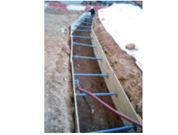
Rasa 1 Tram entibat
