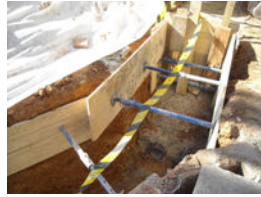
Rasa 1 Tram final entibat 3
