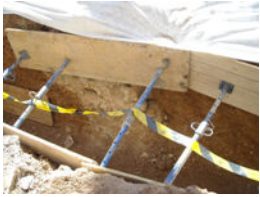
Rasa 1 Tram final entibat 1
