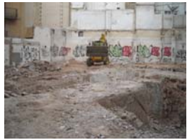
DSCN0269 Vista solar
