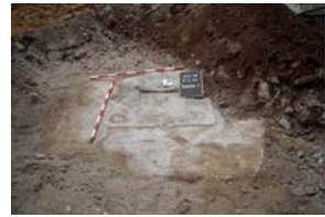
DSCN0344 Rasa 3 Sabata formigó
