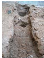
DSCN0291 Rasa 1 Vista general tram Nord
